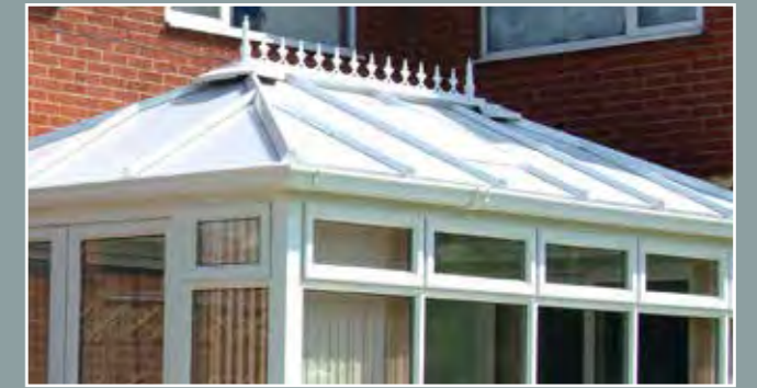
TRADITIONAL CONSERVATORY ROOF
